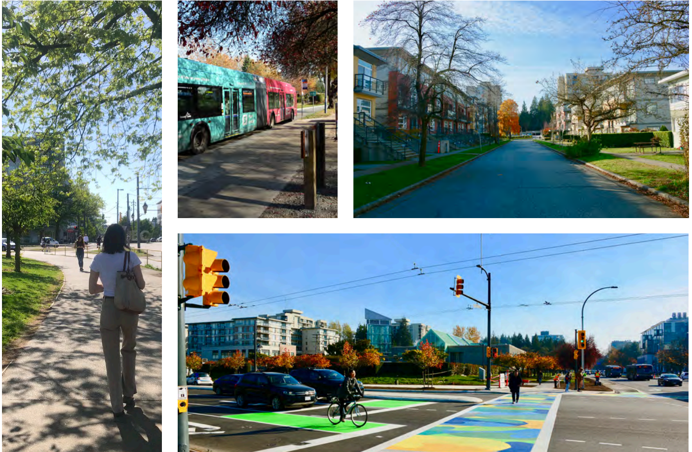
Figure 9: Transportation infrastructure that currently exists in Area D
